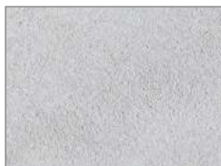
high quality concrete surface inside circle
